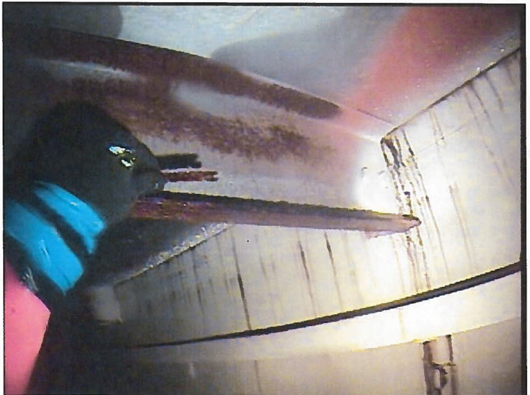
Corrosion truss
