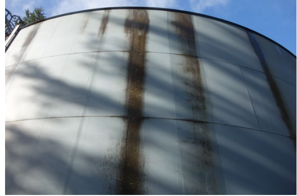
(#4) Exterior Coating Condition #2
