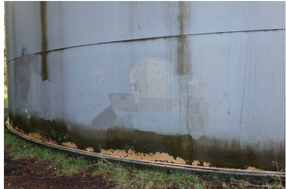
(#10) Exterior Coating Condition #8
