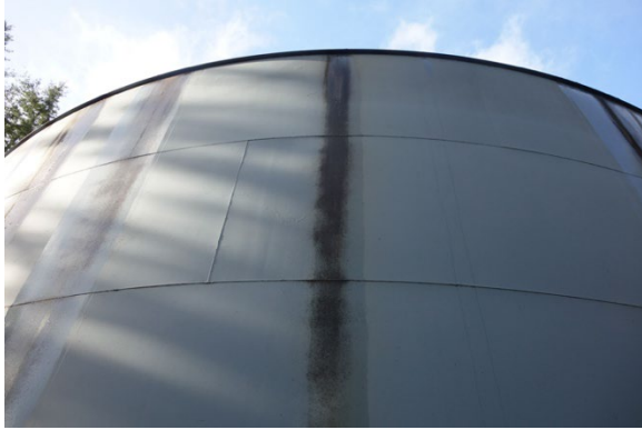
(#1) Exterior Coating Condition #1
