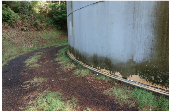
(#11) Exterior Coating Condition #9
