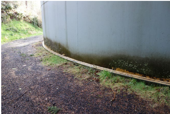
(#7) Exterior Coating Condition #5
