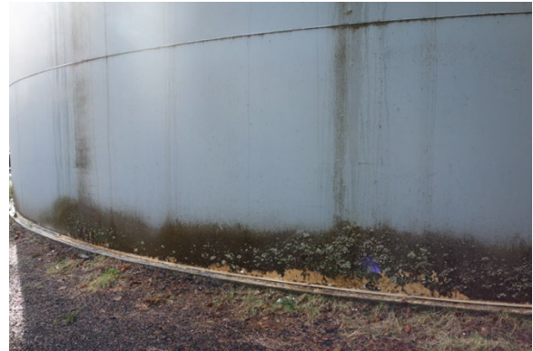
(#5) Exterior Coating Condition #3
