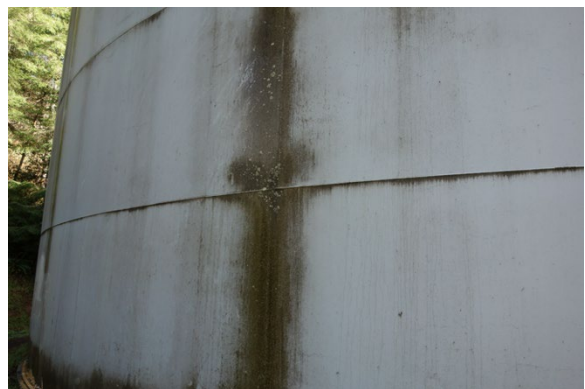
(#12) Exterior Coating Condition #10
