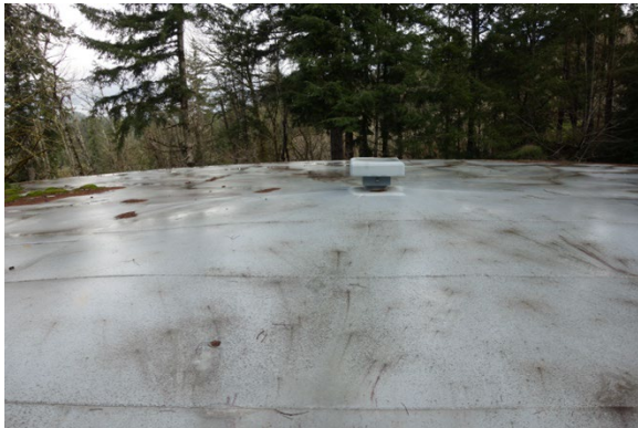
(#20) Roof Coating Condition #3
