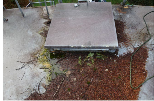
(#22) Roof Access Hatch and Lock
