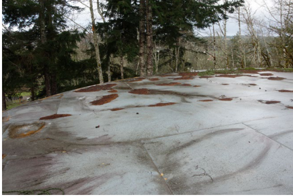
(#19) Roof Coating Condition #2
