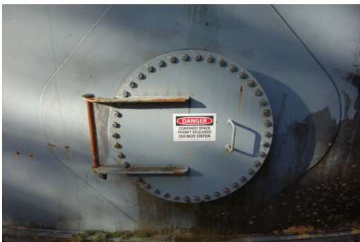
(#44) After Confined Space Entry Placard Installed on Manway
