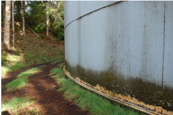
(#14) Exterior Coating Condition #12
