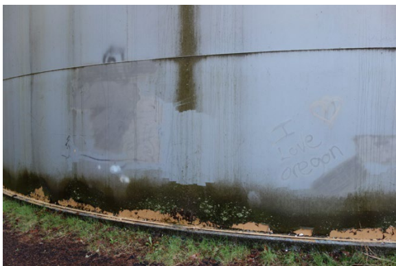
(#9) Exterior Coating Condition #7
