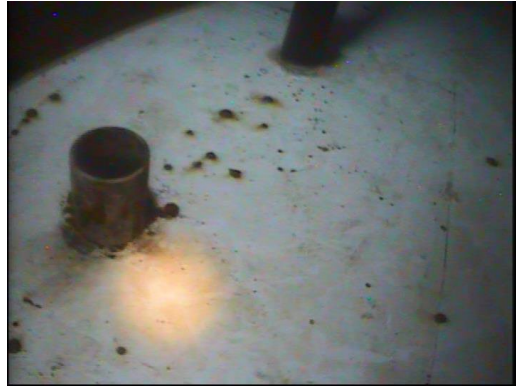
(#34) Inlet/Outlet with Silt Stop
