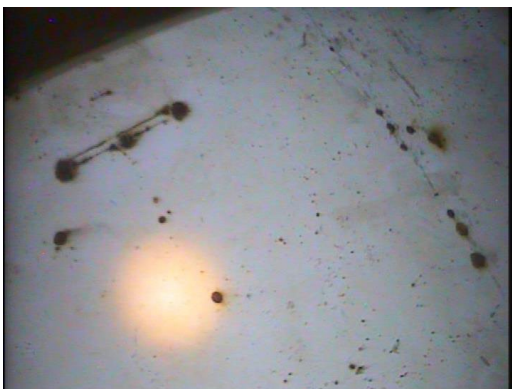
(#33) Float and Wire Guides Broken at Floor Attachment
