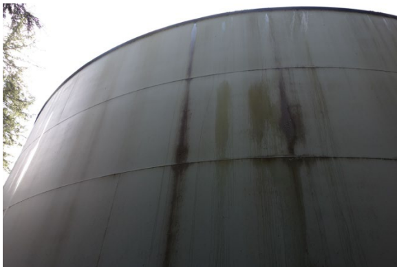
(#8) Exterior Coating Condition #6
