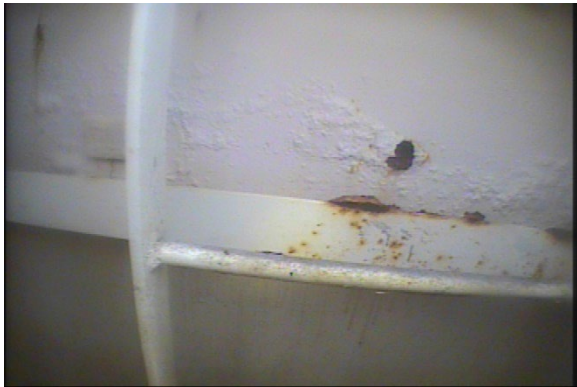
(#26) Interior Ladder Above the Water Line #2
