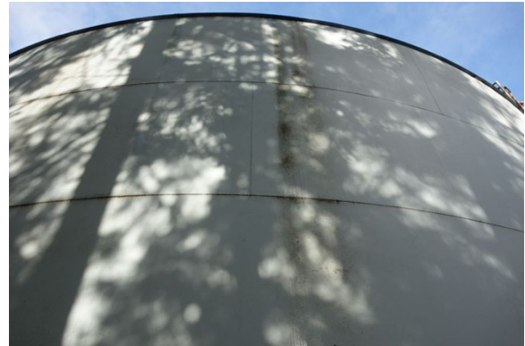
(#16) Exterior Coating Condition #14
