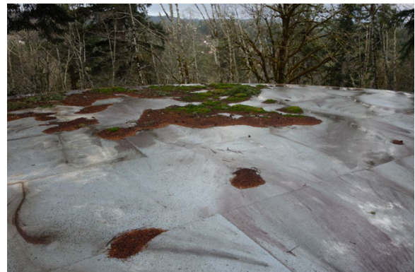
(#18) Roof Coating Condition #1
