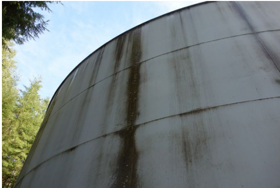
(#13) Exterior Coating Condition #11
