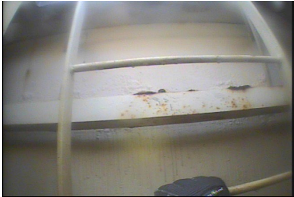
(#25) Interior Ladder Above the Water Line #1
