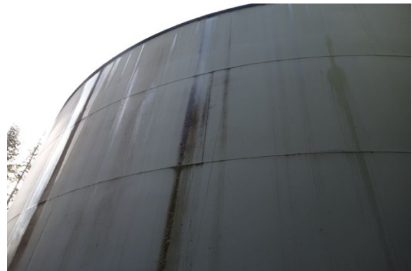
(#6) Exterior Coating Condition #4
