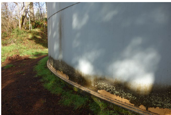
(#15) Exterior Coating Condition #13
