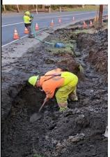
A water line extension of over 900 feet on Business Highway 20 will provide city water services to those near the west junction. This also allows for potential future growth and safety measures by adding fire hydrants along the way.
