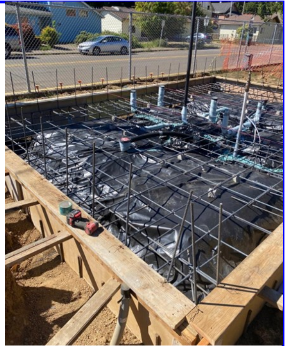
Old tennis court fence being replaced (left); new restroom rebar installation (above).
