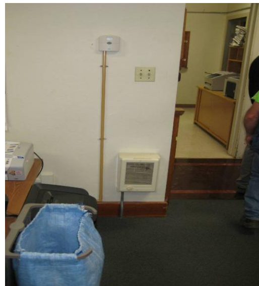
Figure 3.2.1.3 Front Office Heater Controls
