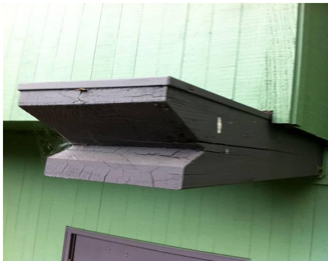
Figure 3.2.4.1A Trim Rotting Beam
