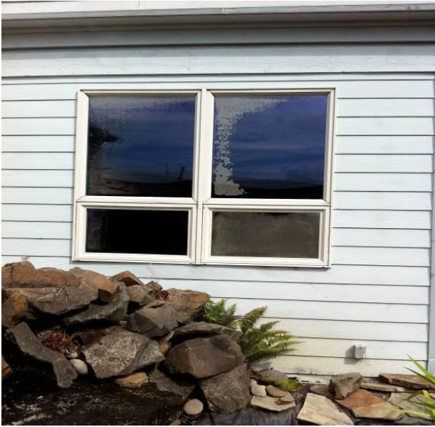
Figure 3.2.2.1A Fogging in Windows
