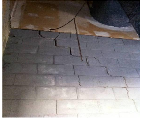
Figure 3.2.5.1B CMU Wall Cracks
