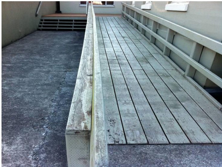
Figure 3.2.1.6 Unsealed Handicapped Ramp with Rot
