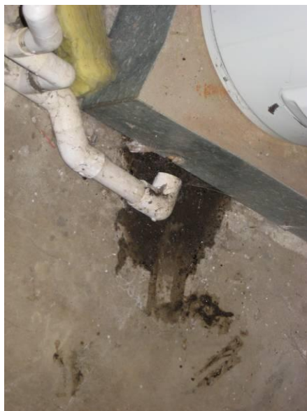
Figure 3.2.4.2A Water Heater Pan Disconnected
