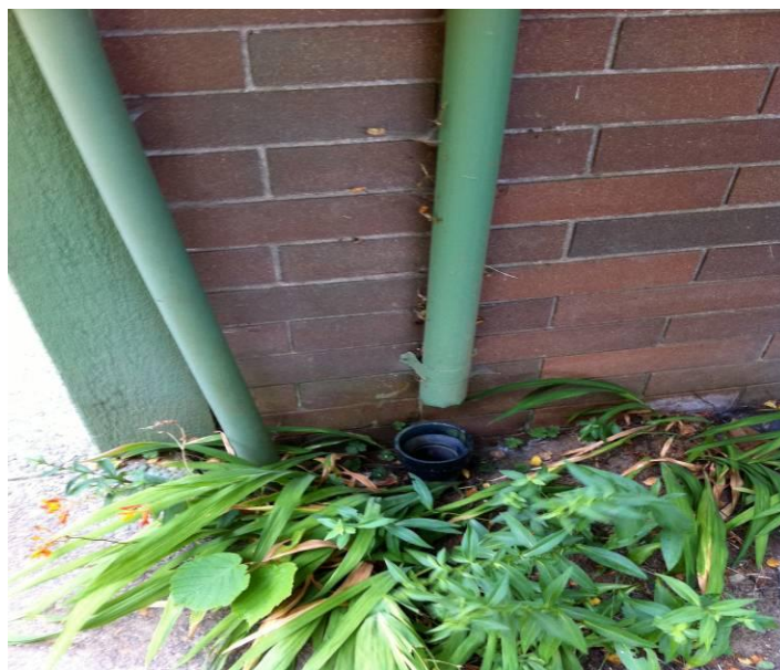
Figure 3.2.4.2B Downspouts Misaligned with Drains
