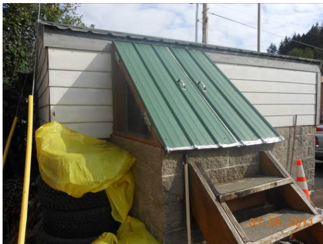
Figure 3.2.2.4 Poor Generator Building Access
