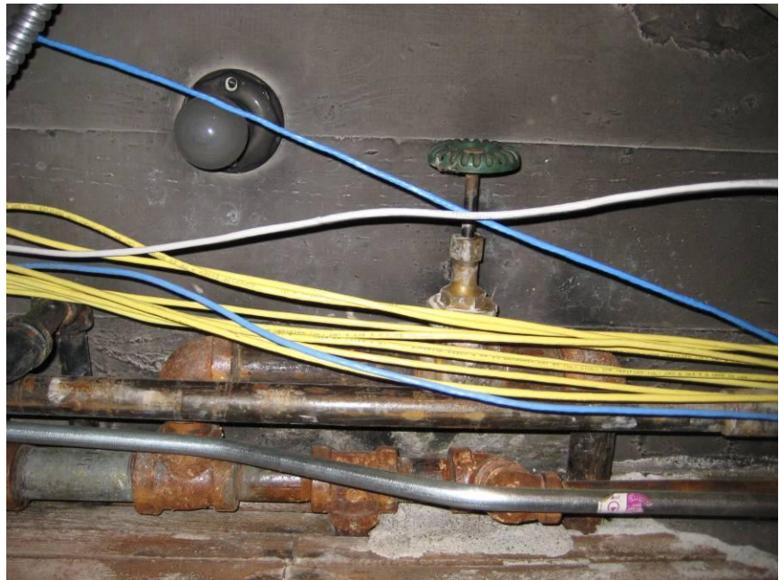
Figure 3.2.1.2 Plumbing Corrosion
