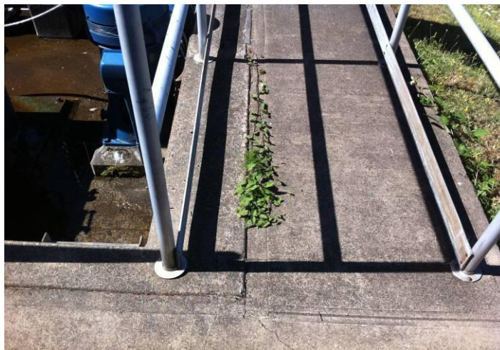
Figure 3.2.7.7 Minor Foliage Problems, Spray and Remove
