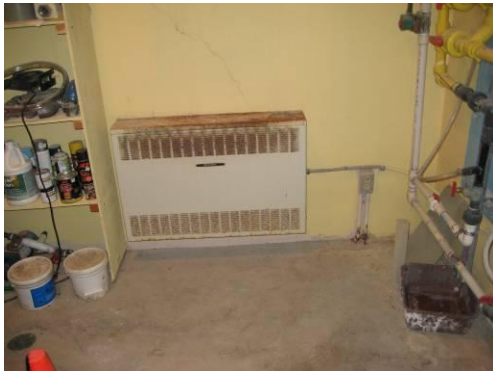
Figure 3.2.7.3 Rusty Heater
