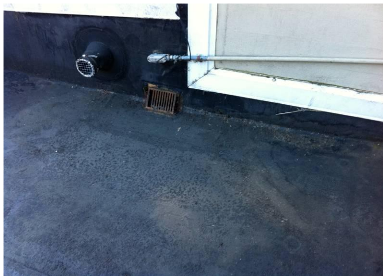
Figure 3.2.8.4 Conduit Blocking Doorway
