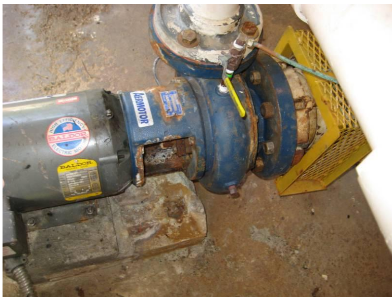
Figure 3.2.5.2 Circulation Pump
