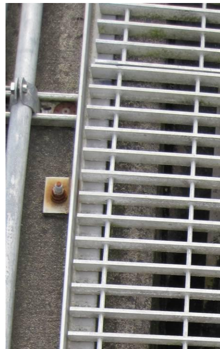
Figure 3.2.8.1 Un-galvanized Anchor
