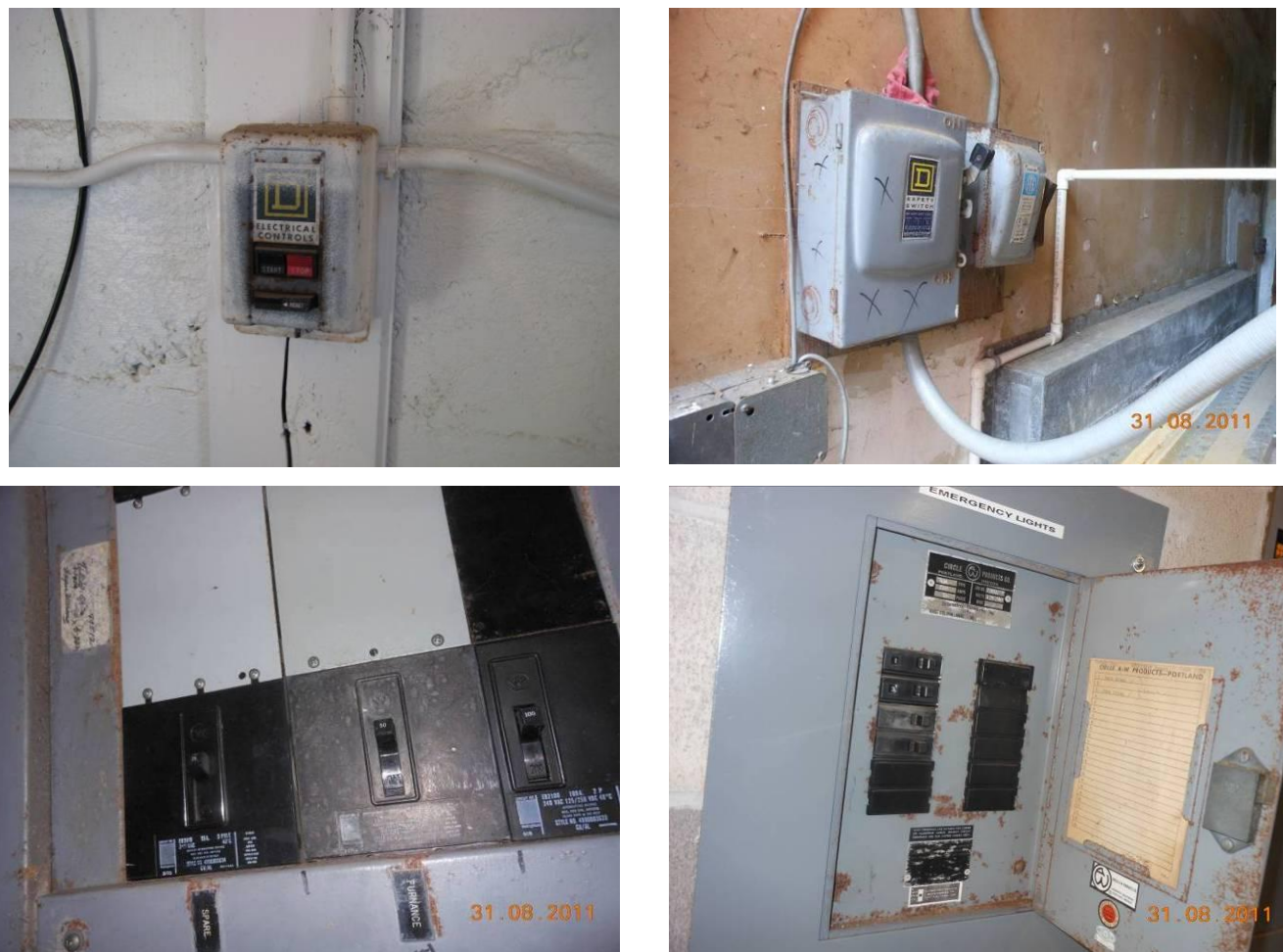
Figure 3.2.5.4 Extensive Electrical Corrosion and Outdated Panels
