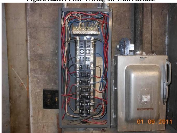
Figure 3.2.1.4B Outdated Pushomatic Basement Panel
