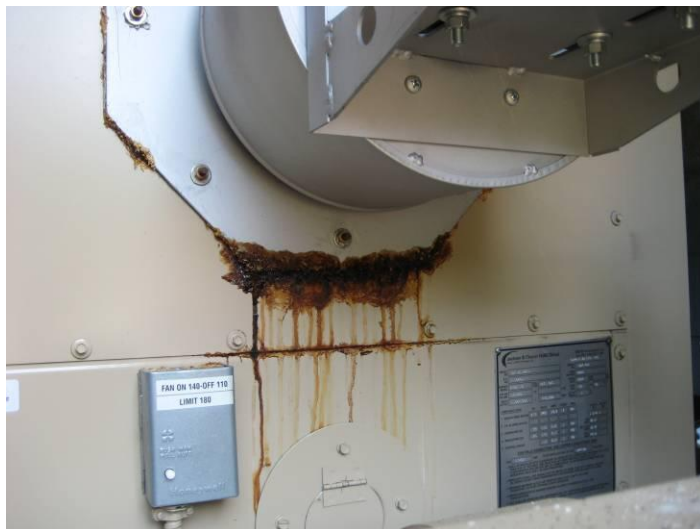
Figure 3.2.5.3 New Furnace Corrosion Evident
