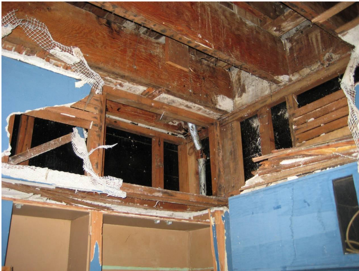
Figure 3.2.1.1C Extensive Water Damage
