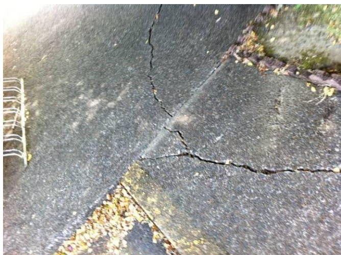
Figure 3.2.4.7A Sidewalk Cracking
