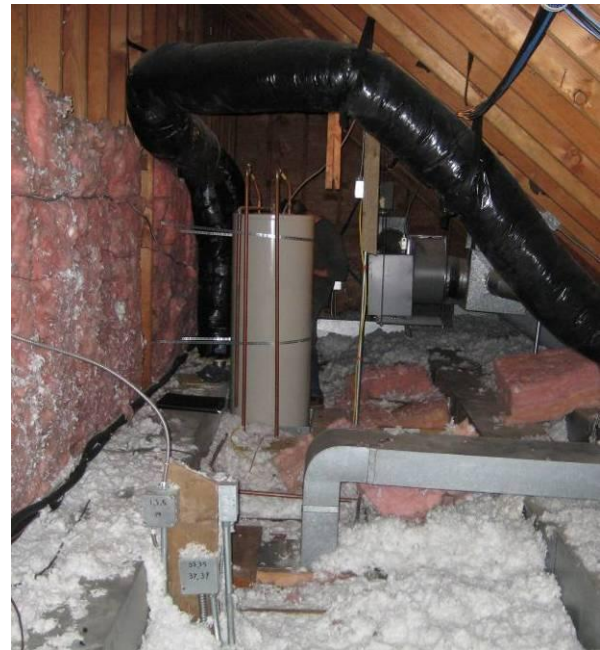
Figure 3.2.2.2 Uninsulated Water Pipes
