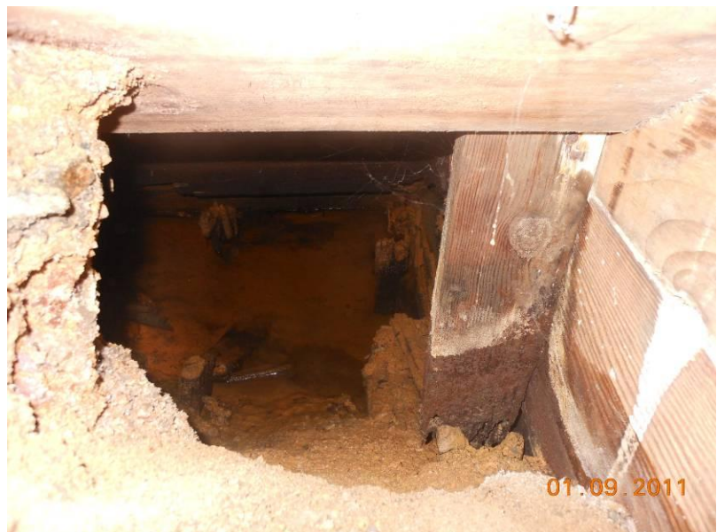
Figure 3.2.1.1A Basement Rot and Standing Water
