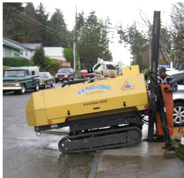
Figure 6.4.3.2 Pipe Bursting Winch
