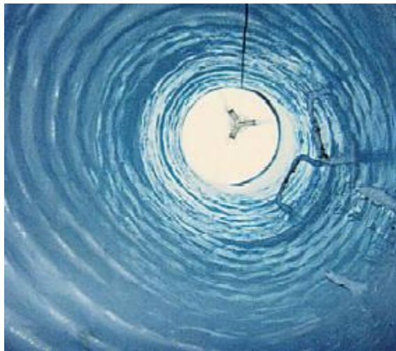
Figure 6.6.1.1 Epoxy Sealed Manhole
