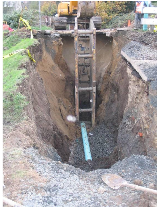
Figure 6.4.1 Open Trench Pipe Construction
