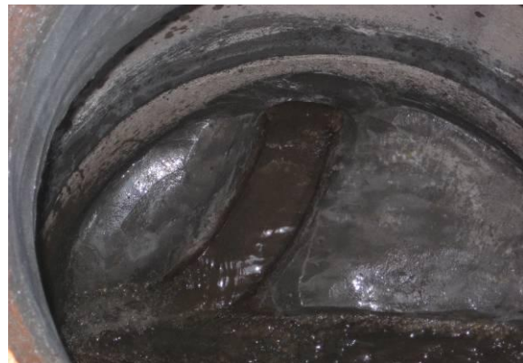
Figure 6.6.1.2 Cementitious Mortar Spot Repaired Manhole
