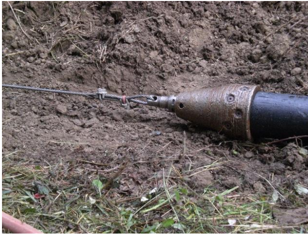
Figure 6.4.3.1 Pipe Bursting Head
