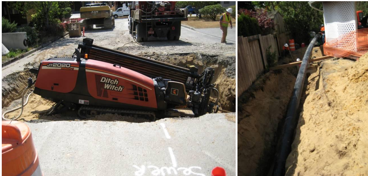
Figure 6.4.2 Pipe Boring
