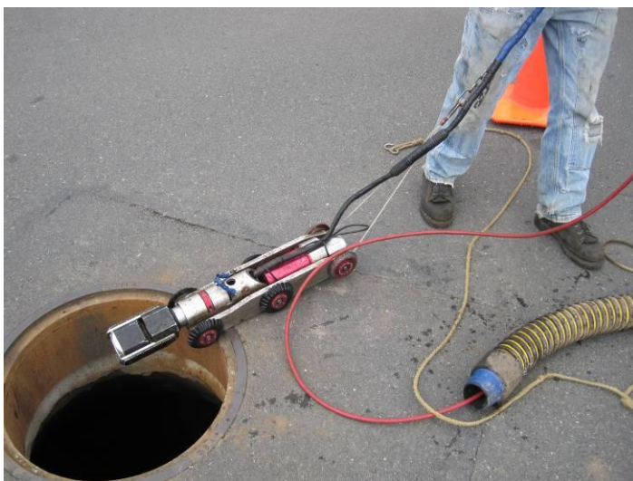
Figure 5.1.2 Televising Camera
