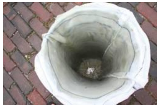
Figure 6.6.2 Manhole Liner
